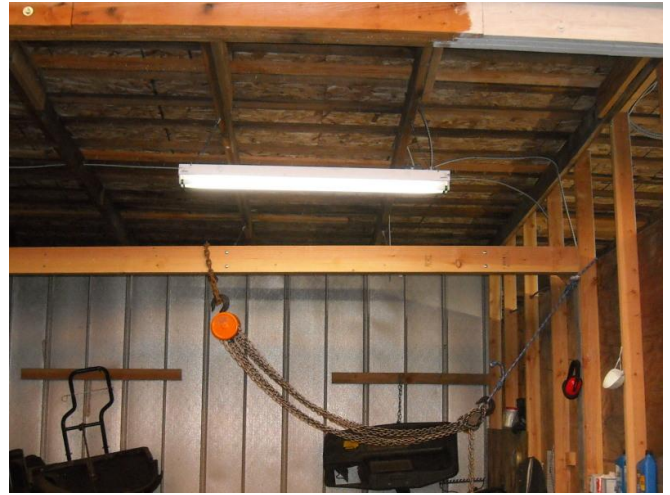
Dual florescent fixture in mower storage area
